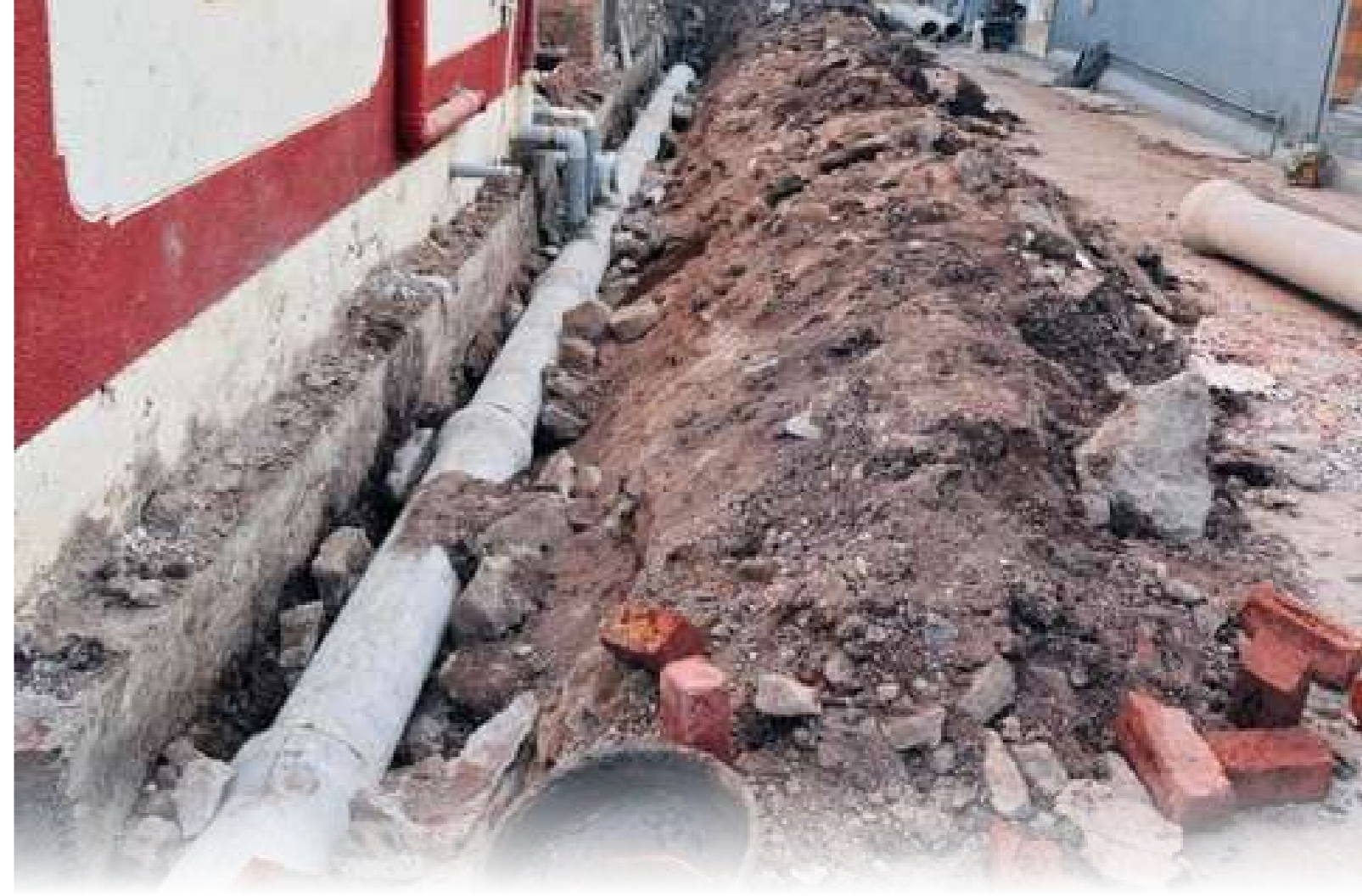
Underground gutters constructed at village Kival. Measurement: 1,500 Mtrs length and 75 number of chambers
